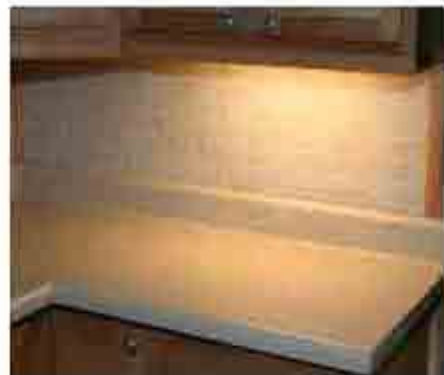
18 in. xenon linear fixture Average illuminance: 204 lux Minimum illuminance: 72 lux Meets recommendation for critical tasks? No Uniformity on counter: 3:1
