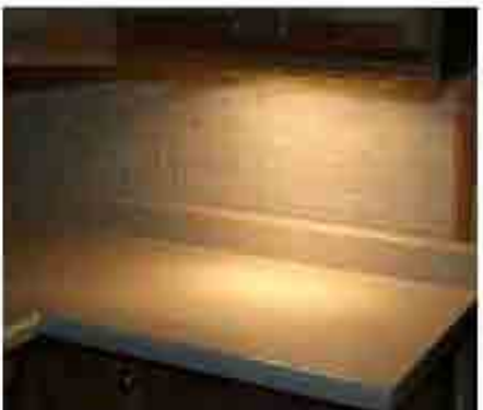
12 in. halogen two puck light bar Average illuminance: 322 lux Minimum illuminance: 90 lux Meets recommendation for critical tasks? Yes Uniformity on counter: 4:1
